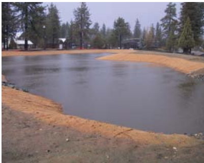
Park Avenue Detention Basin WY2003
