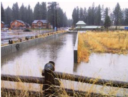
Concrete forebay of Golene Basin, South Lake Tahoe, CA
