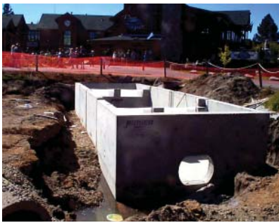
StormFilter® vault construction at Ski Run Marina in 2001
